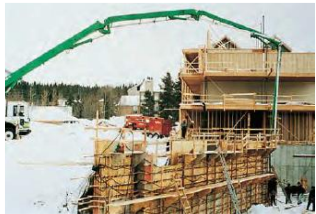
Fig. 8. Hydronic heating system attached to the formwork [10].
