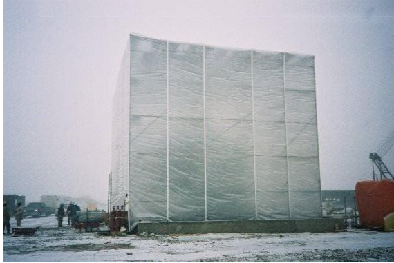
Fig. 5. Unvented fire-enclosed space for curing concrete [5].
